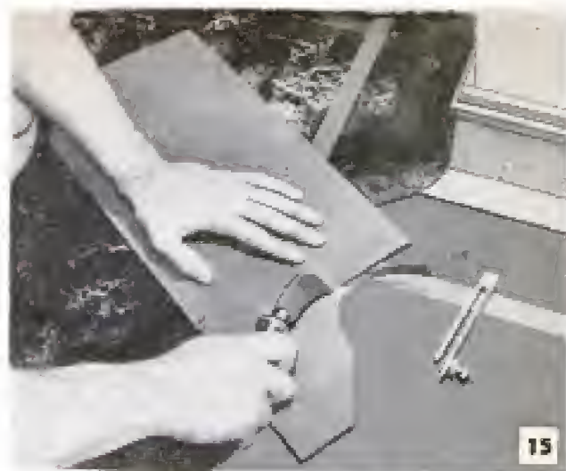
Above, linoleum on self corner is cut at 45-deg. angle down to middle of fillet on outside corners
